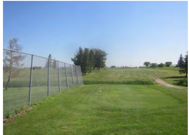
#17 tee with leaning safety fence
