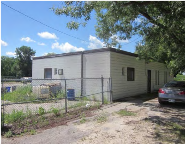
Maintenance shop and yard
