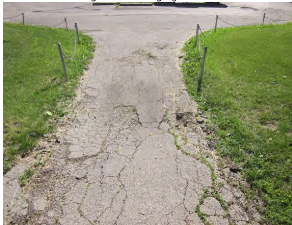
Asphalt paths at entrance to parking lot
