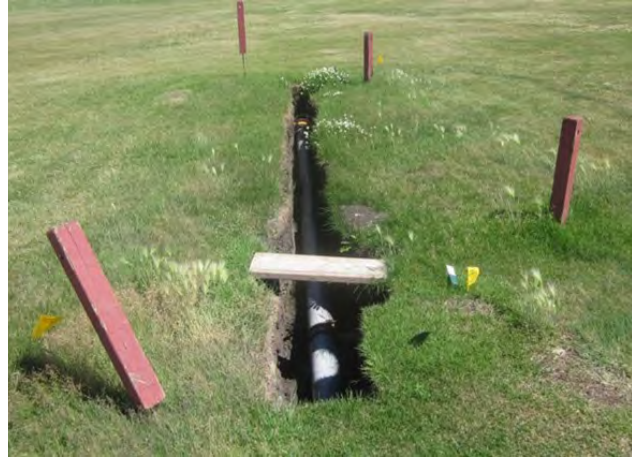
Irrigation main line repair. #1 Gold in front of green
