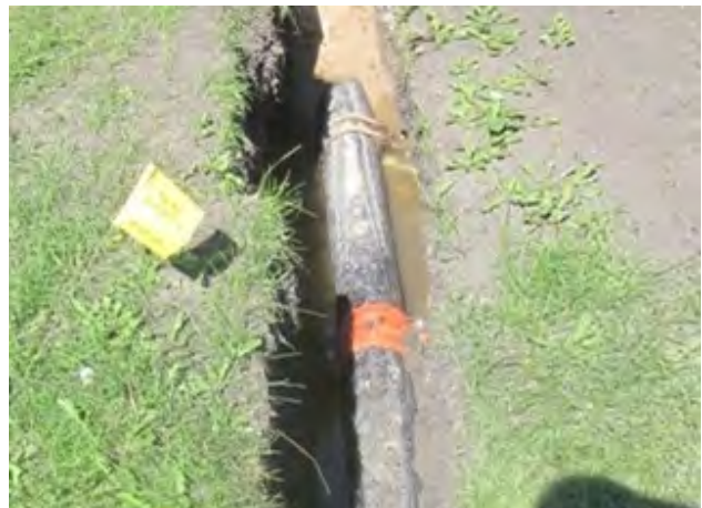
Irrigation break repair – hole #9 on front of tees
